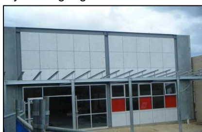
The Multi-purpose Hall under construction
