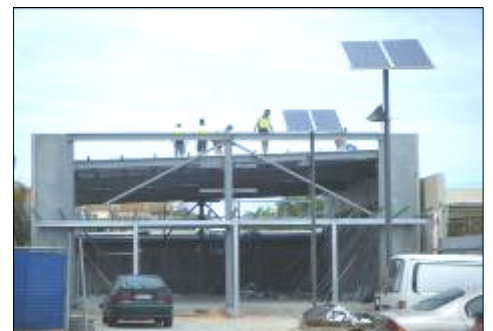
The gym roof is currently being installed.
